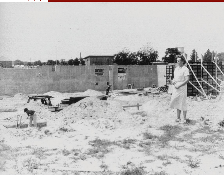
Chaires stands next to the construction site of the campus library.
