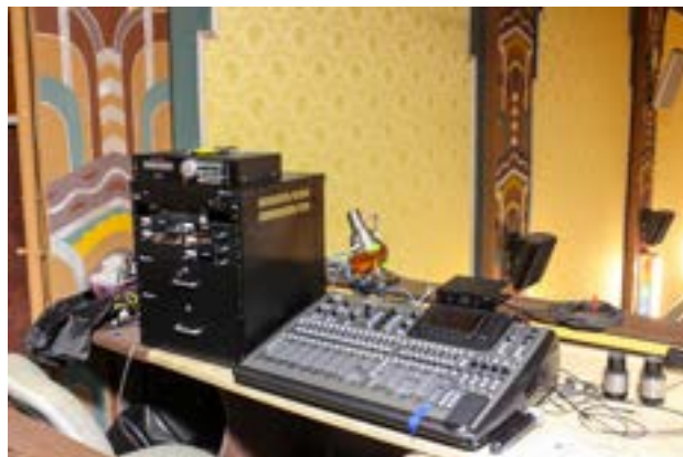
Control room Photo: Madison Ruhl
