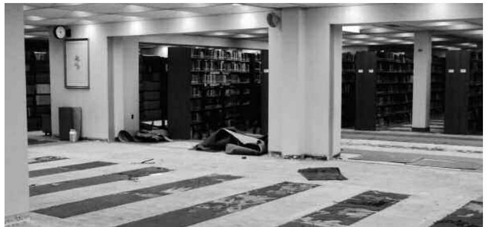
Library recarpeting project
