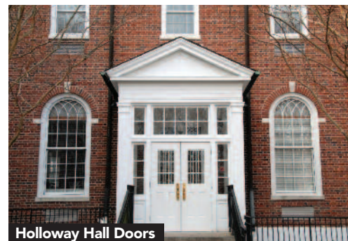
Holloway Hall Doors
