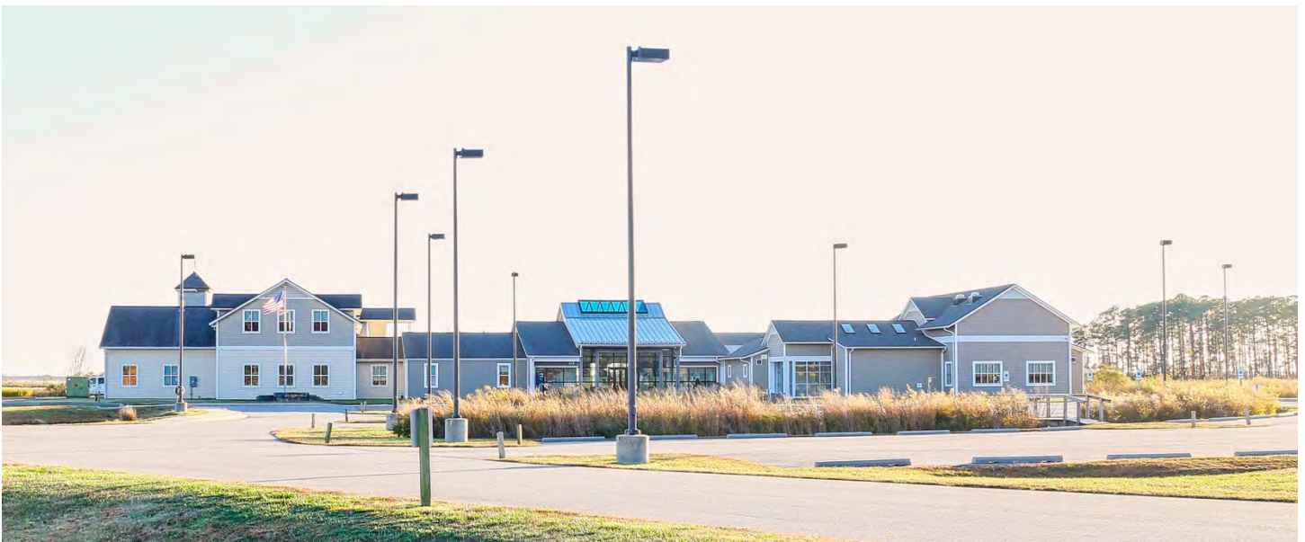
Blackwater Refuge Visitor Center
