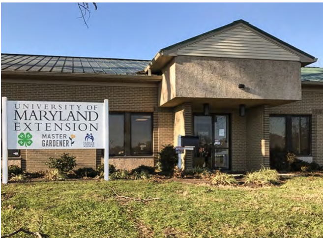
Extension Office, Wicomico Co. Photo: Andrew Southworth
