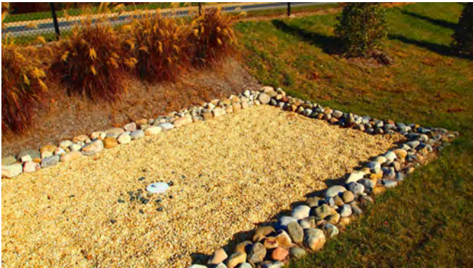
Softball field drainage system Photo: Nathan Voshell
